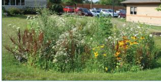
**Figure 1.** Rain garden built to capture rainwater from a parking lot and roof.
