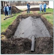
Figure 6. Placing the filter fabric.
