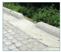
**Figure 4.** Curb cut opening. (Source: USDA, NRCS)
