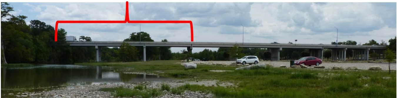
Bracketed area indicates bridge sections where bird exclusion netting will be installed.
